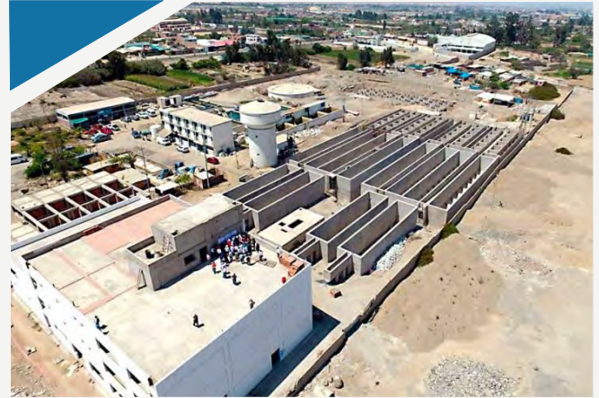
DRINKING WATER TREATMENT PLANT
