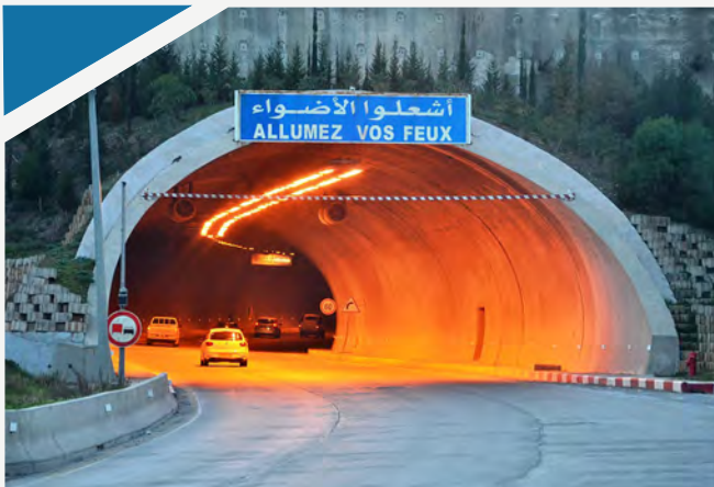
EAST-WEST HIGHWAY TUNNEL
