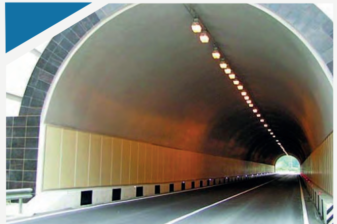
MUMBAI COASTAL ROAD TUNNEL
