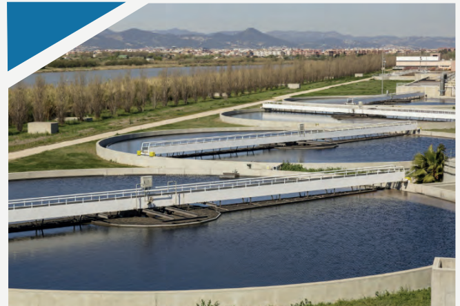
ABRERA PUMPING STATION
